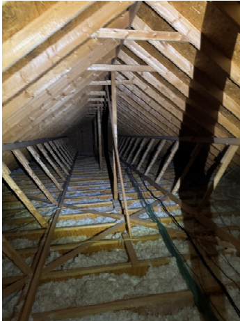
Image of 2x Stick Framing Supported on I Joists at Ceiling at Original Building
